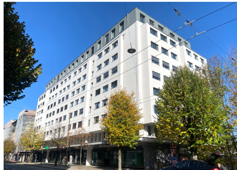
Renovated and extended upwards: PKE property in Fribourg, Rue Jacques-Vogt 1–3 and Boulevard de Pérolles 32–34
